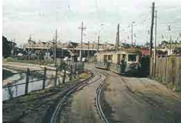
'O' type coupled set of trams Nos.1462 and 1359 on the road to Rozelle Tram Depot, 1958, showing historic fence, and extensive pole gantries for overhead power.
