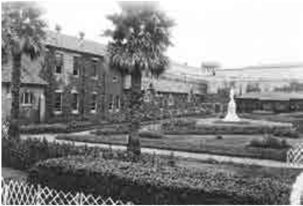
Section of the garden surrounding the (now removed) WW1 memorial. Photograph taken as part of the NSW Tramways Garden 1928-1929.
