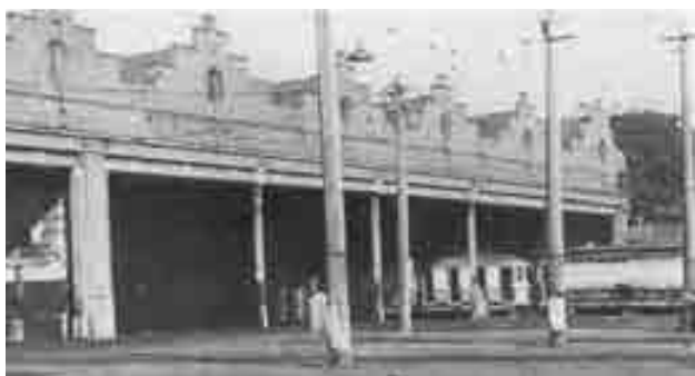
Rozelle tram car sheds showing overhead power gantry, 1948.
