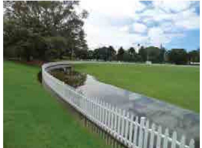
Water pooling after rain event on Jubilee Oval could be captured and treated for later re-use.
